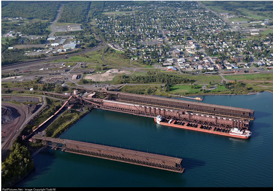
Figure 15-2: Aerial View of the Two CN Operating Docks at Two Harbors, Minnesota
