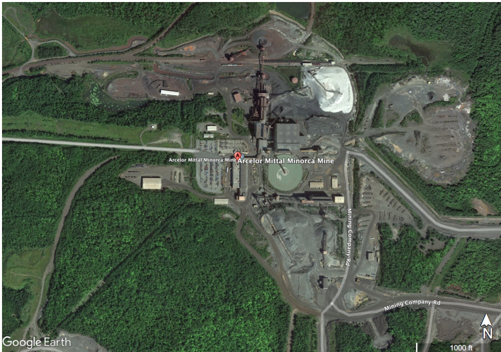
Figure 15-7: Aerial View of Minorca Plant Site
