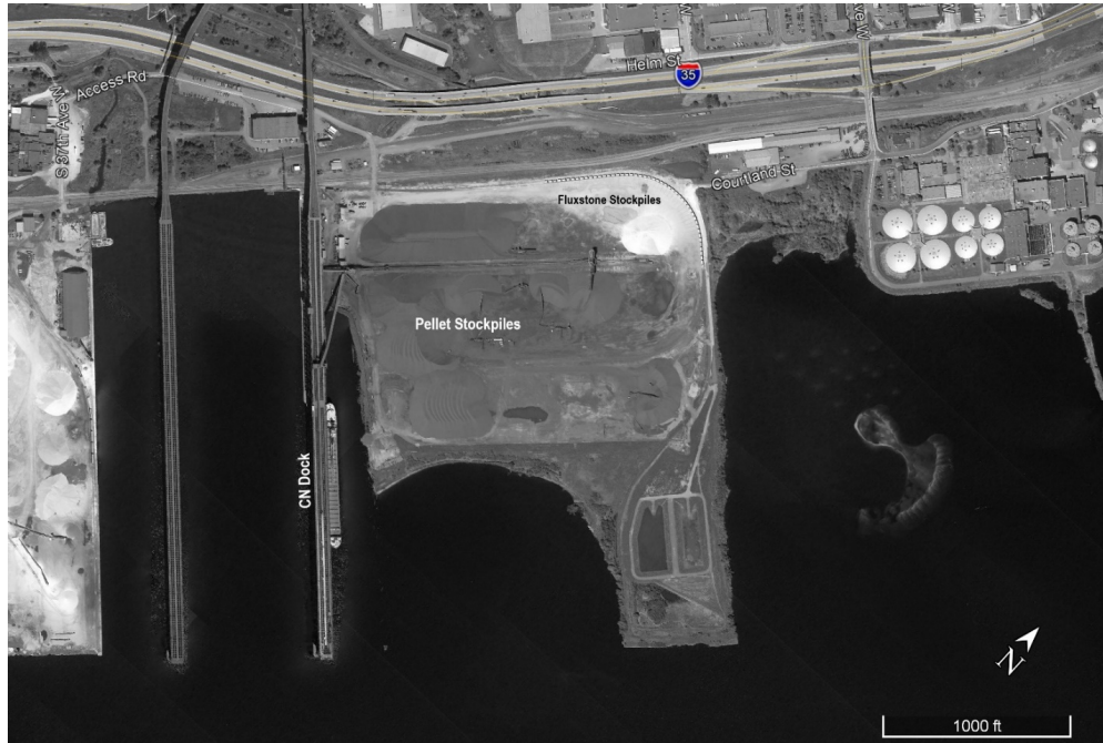
Figure 15-2: CN Dock Facilities - Duluth, MN
